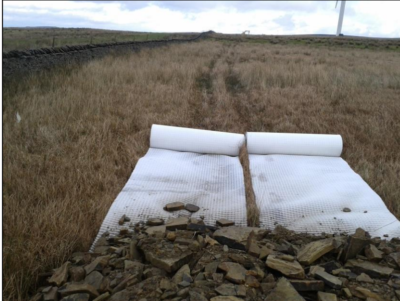
Plate 13: semi-permeable geotextile layer
