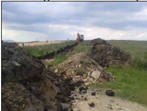
Plate 14: Typical overburden stockpile measures
