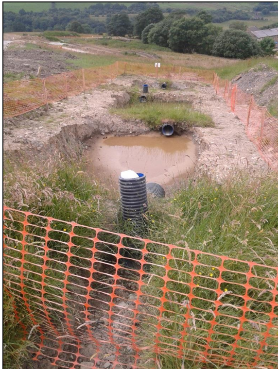
Plate 5: Typical lagoon and flocculent station
